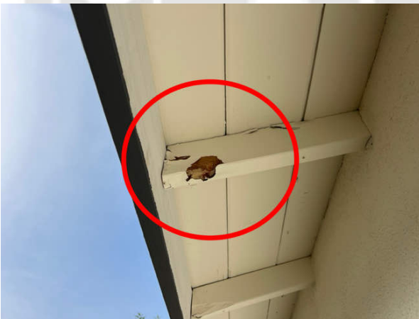
EXTERIOR WINDOWS WINDOW TYPE 61: Aluminum frame thermal pane windows.
