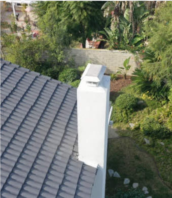
CHIMNEY STORM CAP & SPARK ARRESTOR 64: Storm cap and spark arrestor were present.
