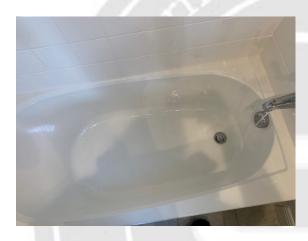
**251:** The diverter valve is a component used to divert water from the tub spout to the shower head. A fair amount of water was still flowing through the tub spout when the diverter valve was actuated. This is an early sign of failure. Replacement recommended.
