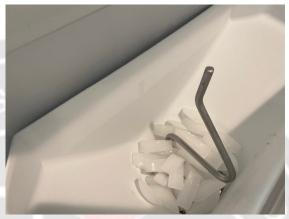
**176:** The refrigerator showing signs of deferred maintenance. Cleaning needed. Fresh food refrigerator temperature was 60° wind tested. This is not a suitable temperature. Temperature should range between 30 and 36°. Consult with an appliance repair man for complete evaluation if adjusting the temperature does not help.
