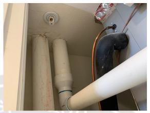
**95:** Moisture damage was noted at the vent pipe. Recommend further evaluation and repair by a licensed HVAC technician.
