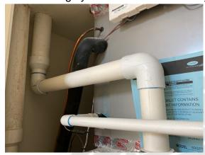
**109:** Because of the close proximity to the return air register. It is strongly recommended that the door to the heating system be properly sealed. This will prevent air scavenging from the furnace closet.
