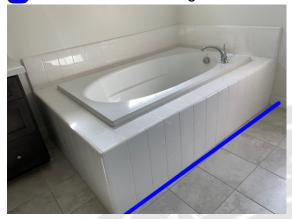
**228:** Damage and cracked tiles were observed on the day of inspection. Damaged or cracked tiles can lead to water infiltration and concealed mold. Repairs needed.
