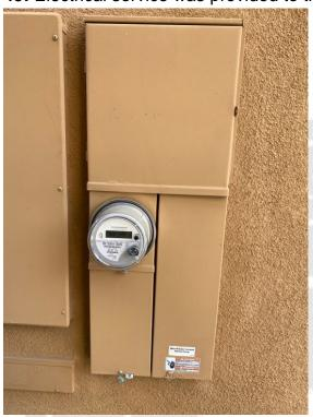
**46:** Electrical service is provided to the home via underground service conductors. These service conductors are not inspected as they are buried below grade.
