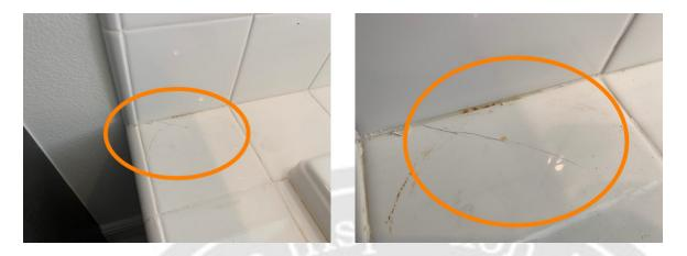
**229:** Deficient and or missing tile grout was noted. This condition can lead to water infiltration and concealed mold. Repairs needed.
