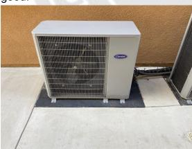
**102:** AC condenser was sitting on a pad. However, the pad should have been installed above concrete grade level. Installing the condenser at grade level can lead to rust and corrosion. Consult with an HVAC contractor for correction.
