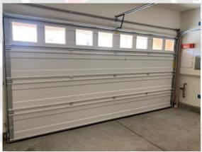
131: Sectional rollup doors have a unique set of safety concerns. Pinch points and operable cables can cause severe injury. The door should not be operated while individuals or objects are in close proximity to moving components.
