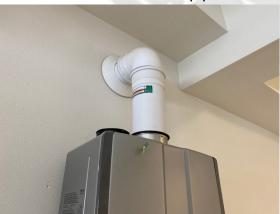
**81:** The wall flange at the exterior of the home was not properly sealed to the structure. Subject to water intrusion. Repair needed.
