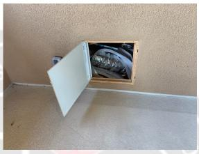
**290:** The attic access hatch was damaged or broken. Additionally there are wires and ducting obstructing the hatch from being opened completely. These conditions prevent the attic area from being inspected.
