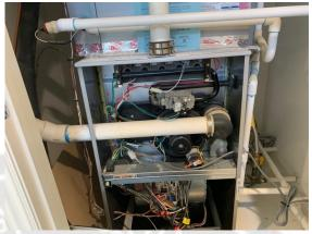
**93:** Because of the close proximity to the return air register. It is strongly recommended that the door to the heating system be properly sealed. This will prevent air scavenging from the furnace closet.
