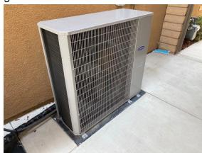
**118:** AC condenser was sitting on a pad. However, the pad should have been installed above concrete grade level. Installing the condenser at grade level can lead to rust and corrosion. Consult with an HVAC contractor for correction.
